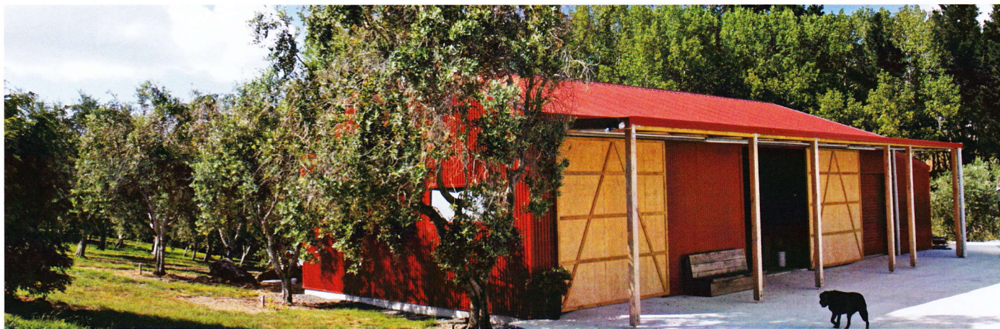
The Matakana co-op recently built a shed on one of the properties, providing a central point for oil storage, bottling and packaging.
