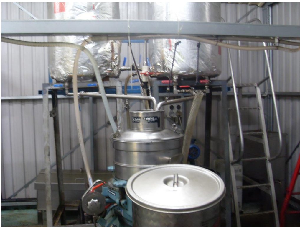
Separator to oil holding tanks
