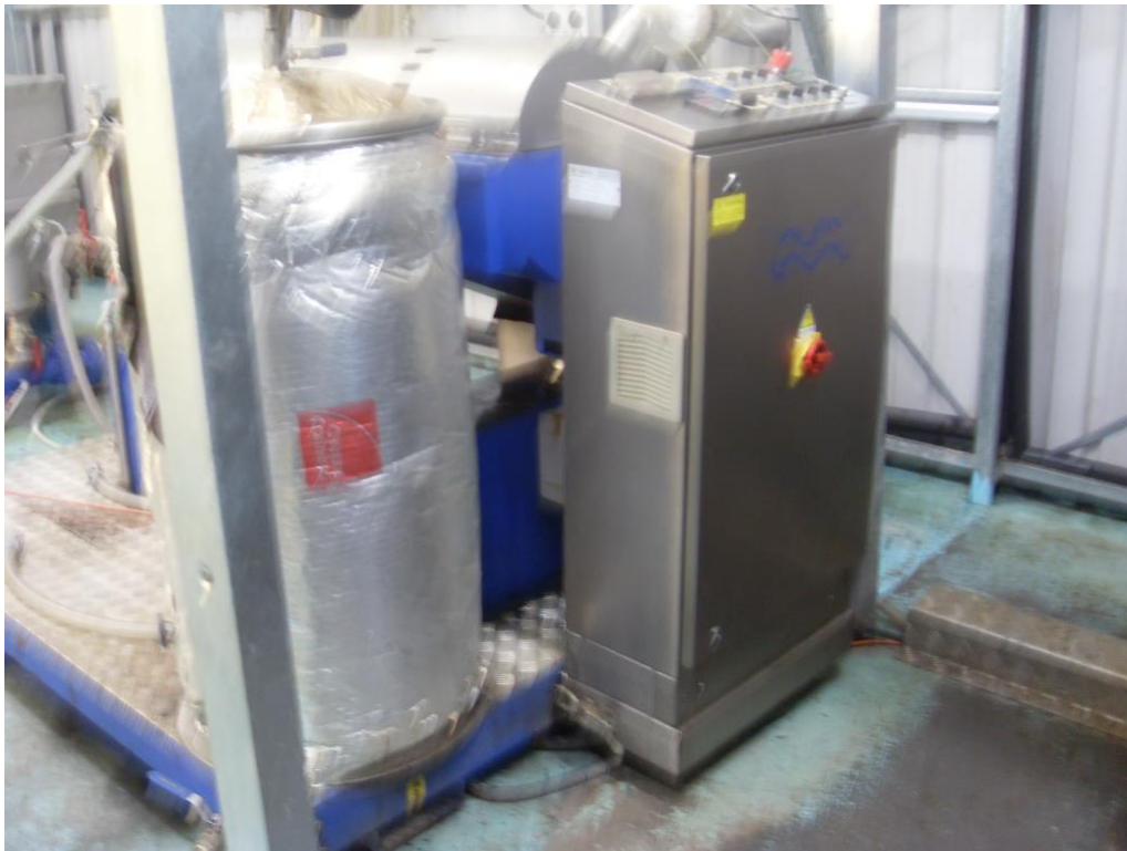
Decanter control box
